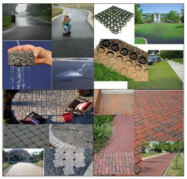
Figure 3: Examples of Permeable Paving
